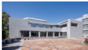
(Ohashi) Renovation of the Multi-purpose Building Completed in fiscal 2023
