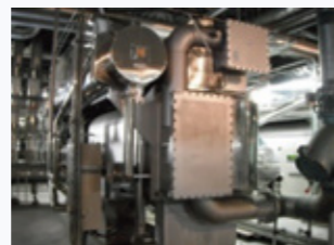
Absorption-type refrigeration unit powered by city gas and heavy oil
